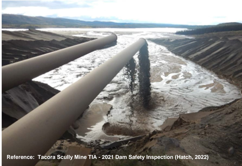
Figure 4-3: Tacora's Existing Thickened Slurry Tailings Pipeline Discharge
