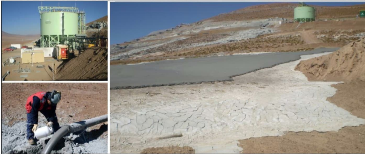
Figure 4-10: Example Paste Tailings Pipeline Discharge
