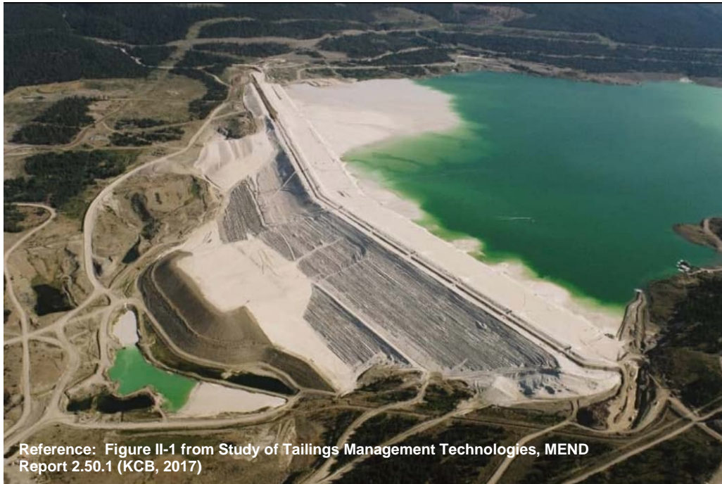
Figure 4-4: Example Slurry Tailings Impoundment Using Earthen Dam Structures
